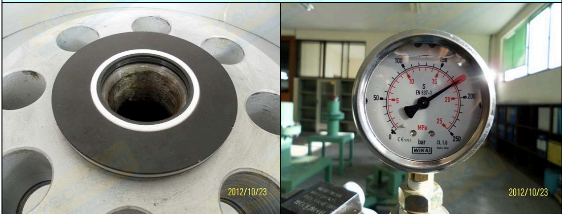
Hydraulic Pressure (180kg/cm 2 ) : No Leakage
